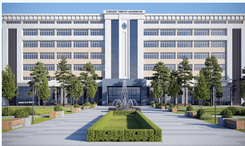
FIRST TASHKENT STATE MEDICAL INSTITUTE, UZBEKISTAN
